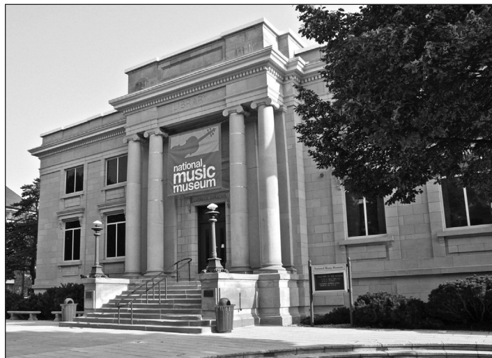
The National Music Museum, University of South Dakota campus, Vermillion, South Dakota, looking northeast (June 19, 2016).
